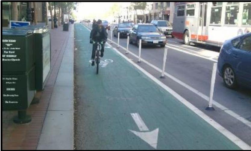
**Typical separated bike lane with vertical buffer on roadway**
